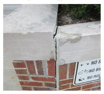
The sealant joints on the brick walls, window and door perimeter, and pavement are in poor condition or missing.
