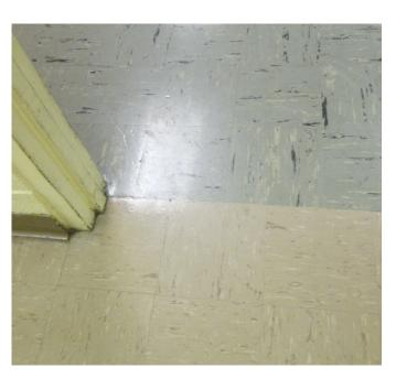
Classroom 11 on the first floor appears to have a persistent moisture infiltration through the VCT flooring. According the classroom teacher, mold has been previously scrubbed off the surface. However, it appears that it is again starting to grow again.
