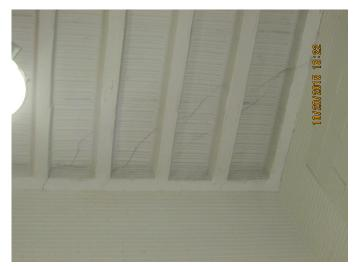
The Wrestling Training room 180 on the second floor is in poor condition with damaged plaster walls and ceiling tiles.
