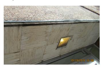
There is wood frame structure addition located on the southwest corner just of the Receiving area. The wood siding, soffit and fascia boards are badly stained and discolored. It appears that some of the boards are starting to rot.
