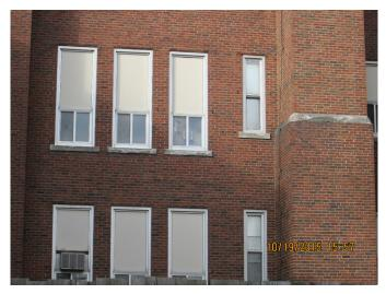
The building addition located at the southwest corner has an aluminum curtain wall system that is in poor condition. The wall system has uninsulated single glazing and the sealant joints are missing or deteriorated. Some of the window panels appeared to have been blocked off with insulation in an effort to conserve energy.
